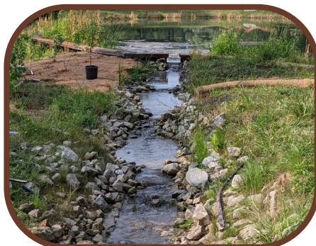
Modified outlet allowing fish passage
