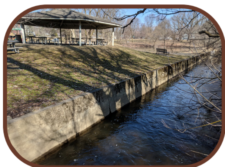
Concrete wall channelizing creek
